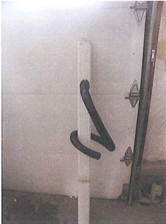
Diverter Installed in Sample Downspout
