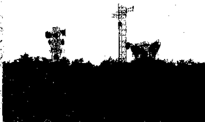
Cell phone towers have become a common feature in the built environment.
